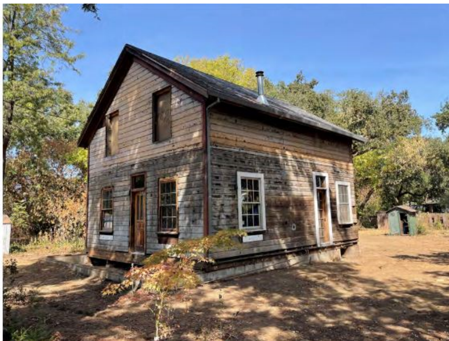
Original two-story structure after removal of additions and wood shingles (R. Claes, September 2021)
