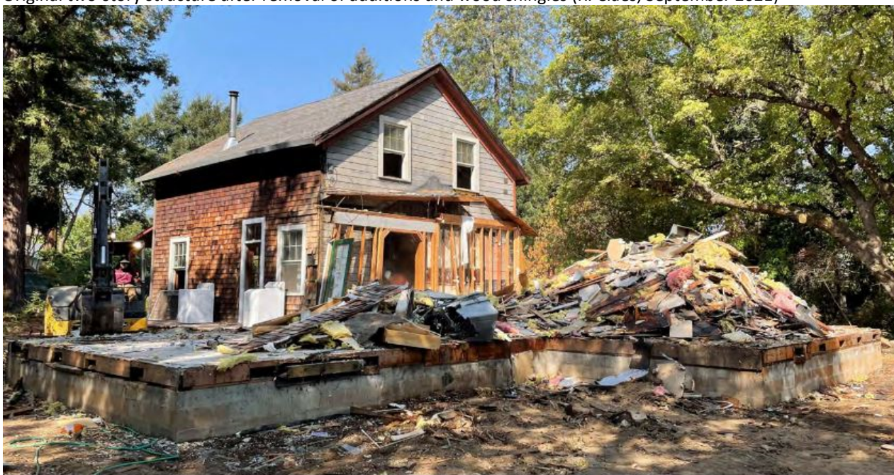
Removal of non-historic addition (east elevation), in progress (R. Claes, September 2021)
