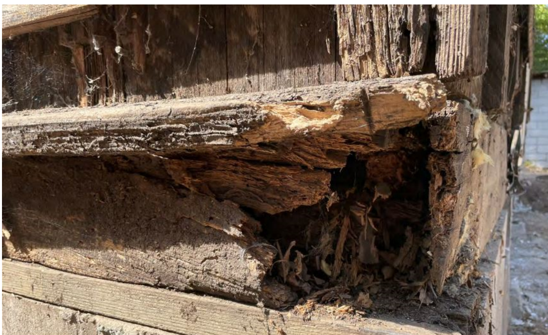
Typical deterioration due to water infiltration (R. Claes, September 2021)
