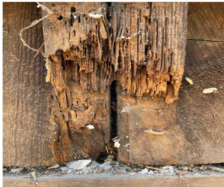
Rotted Structural Framing Due to Excessive Water Infiltration
